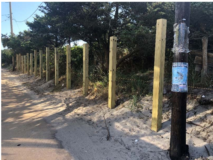
BOTTOM LEFT 2: Photos depicting areas where post installation for retaining wall began. Note that trees and utility poles were avoided.
