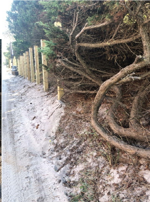
BOTTOM LEFT 2: Photos depicting areas where post installation for retaining wall began. Note that trees and utility poles were avoided.
