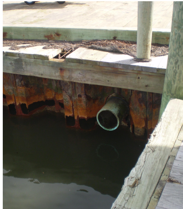
Installation of backflow prevention devices on existing outfalls
